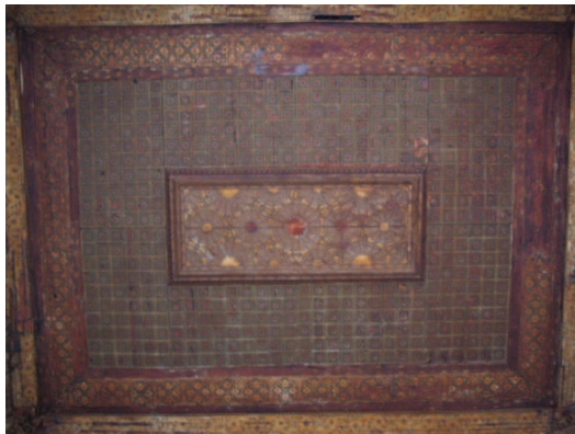
Figure 33. Iwan ceiling, Rami, 2006
