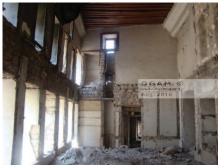
Figure 14. Room of AJEK-PASH 20/Aug/2016
