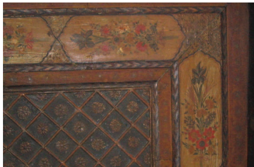
Figure 29. rectangular qa’a in the north east
