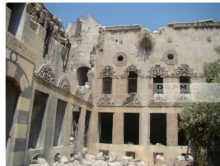
Figure 15. Room of AJEK-PASH 20/Aug/2016
