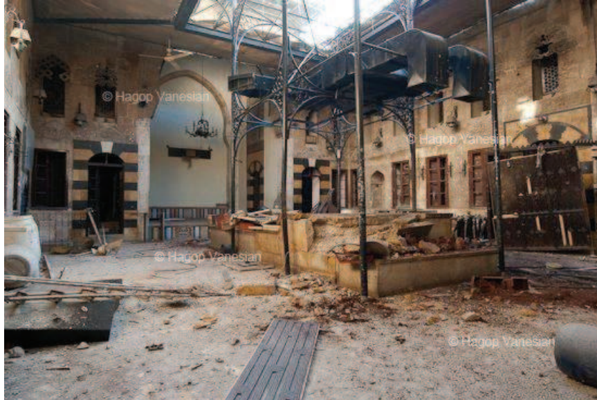
Figure 31. Damages in the Wakil House, northern courtyard, Hagop Vanesian
